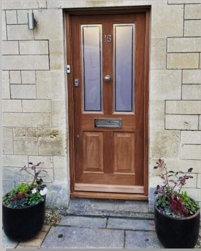
Solid Sapele timber replacement door and frame...
