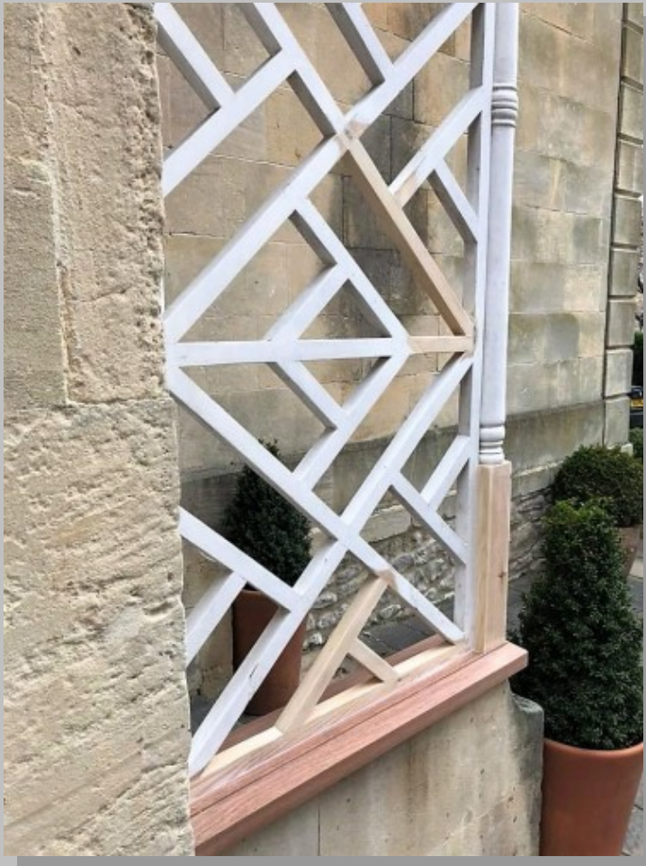
Repairs to this Porch Trellis support
