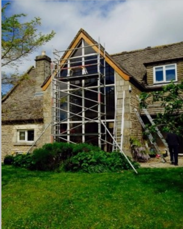
Replacing fascia boards
