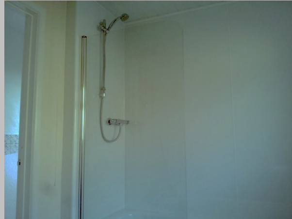
Bathroom wall panels
