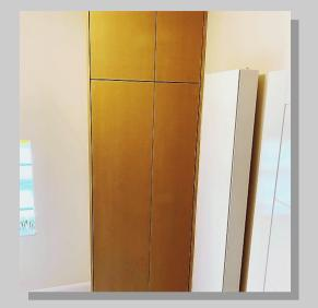
Loft conversion second fix and eave (storage), modern flush push to open finishes. External bookcase storage and boiler housing to match with removable internal shelving. Filled, sanded and sealed ready for the decorators to work there magic.
